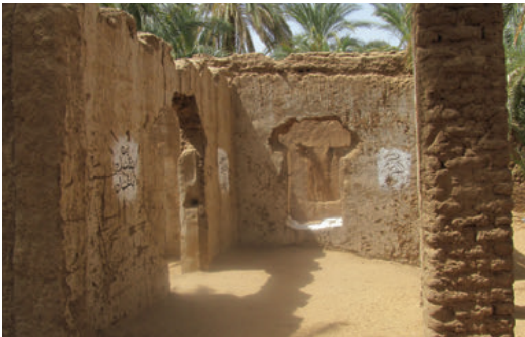
Fig. 5 Karmakül (23.02.18), fragment of the residence of a former ʿumda – the inner part. Photo by Andrzej Leligdowicz
