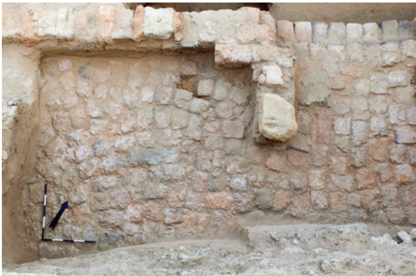
Fig. 9 The bricked pavement around the lower church. Photo by Michał Dzik
