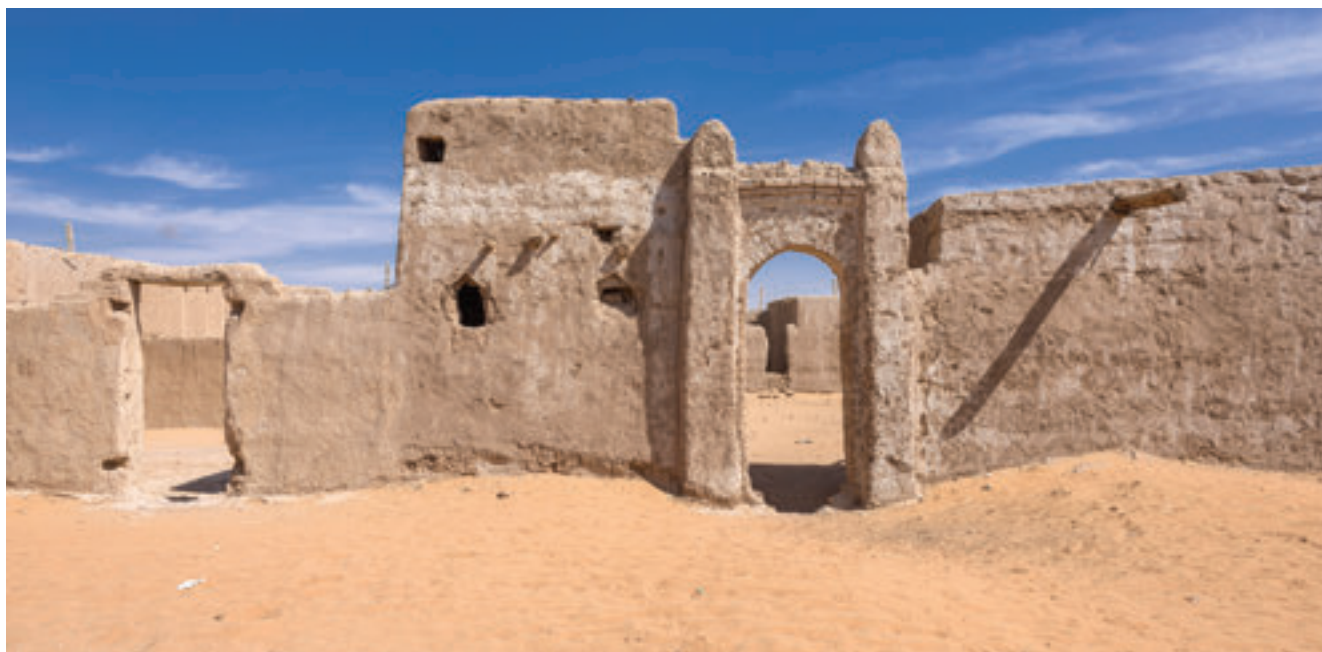
Fig. 13 Bukubūl (9.12.2017), entrance to an abandoned old building. Photo by Andrzej Chojnacki
