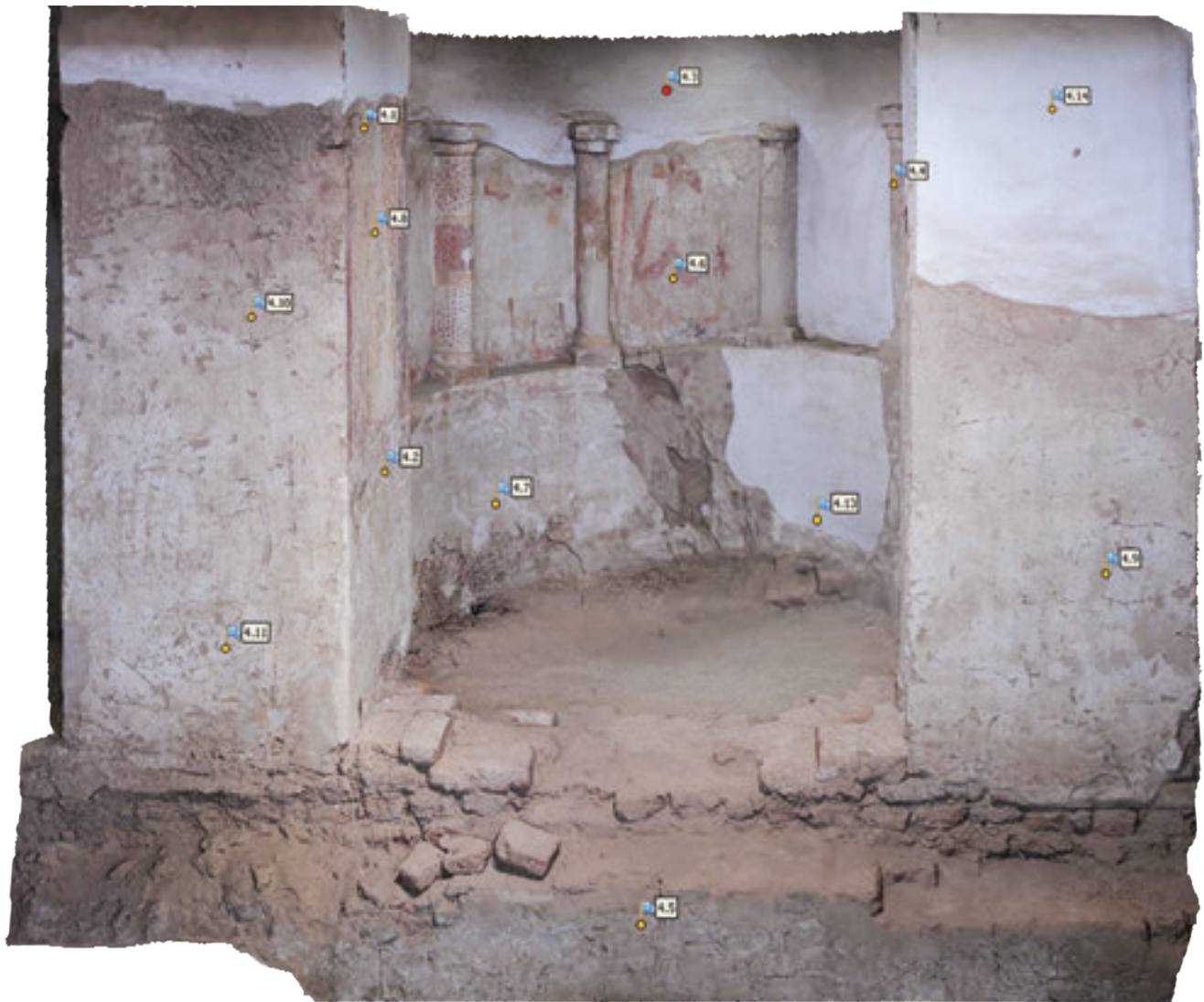
Fig. 17 Example of distribution of natural control points in Chapel 4, a small-size object
