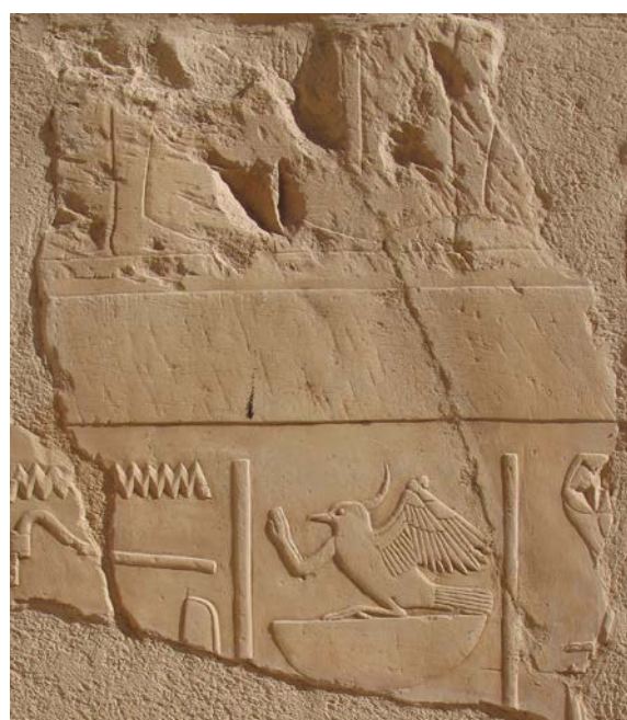
Fig. 41. Traces of chisel from the time of preparation of the wall (phot. J. Iwaszczuk).
