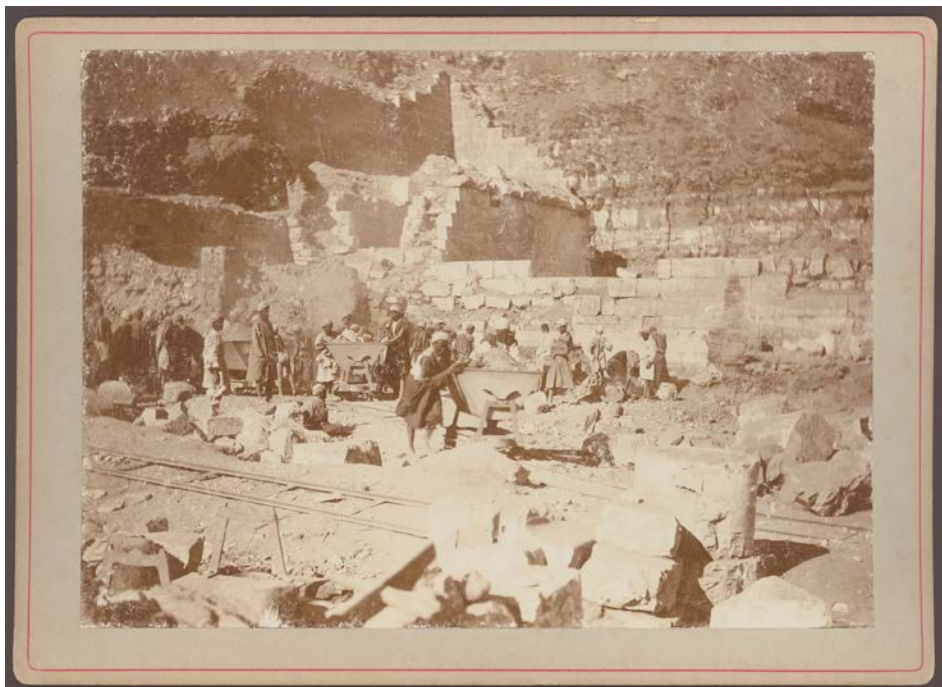
Fig. 12. Excavations of Naville in the north part of the Upper Courtyard with use of a line of railroads (© Museum of Art and History, City of Geneva, inv. no. Naville_HM_0051).
