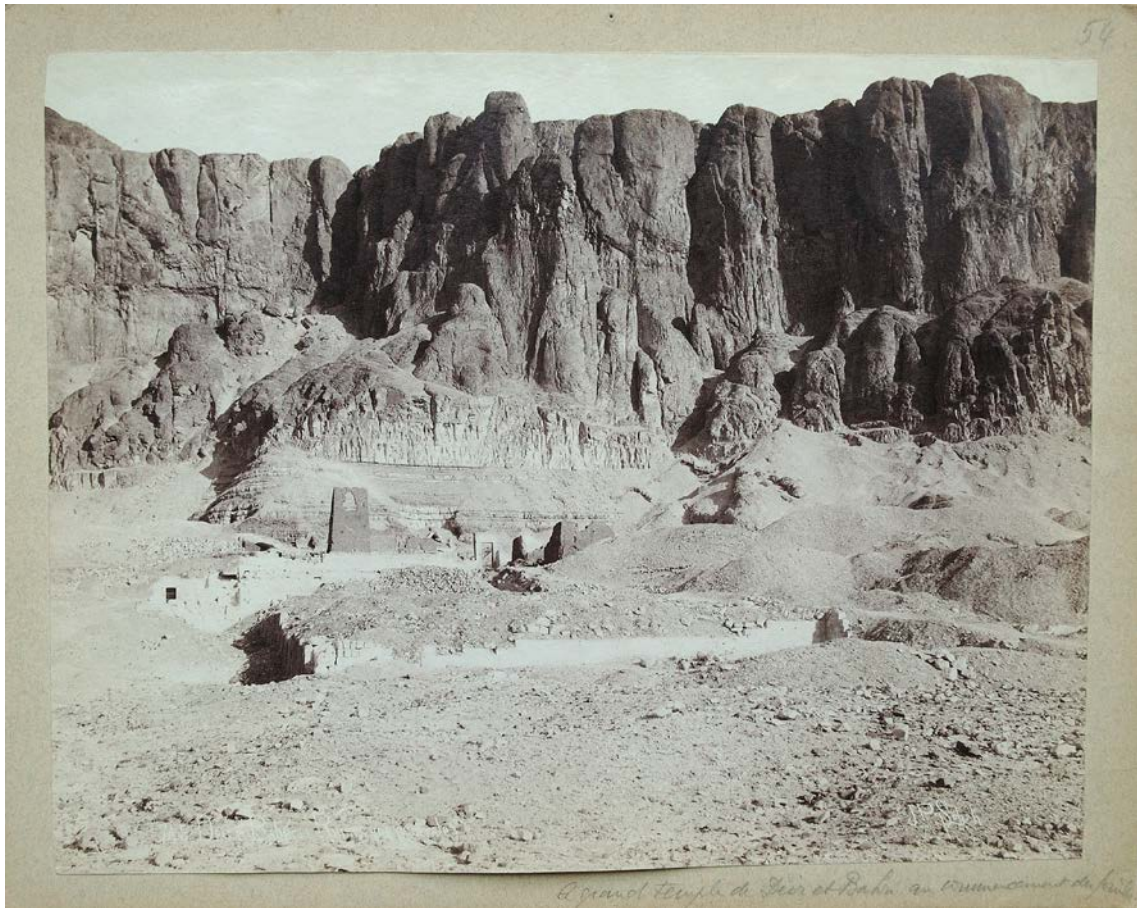
Fig. 13. View on the temple of Hatshepsut from the south-east (© Museum of Art and History, City of Geneva, inv. no. Naville_HM_0064).
