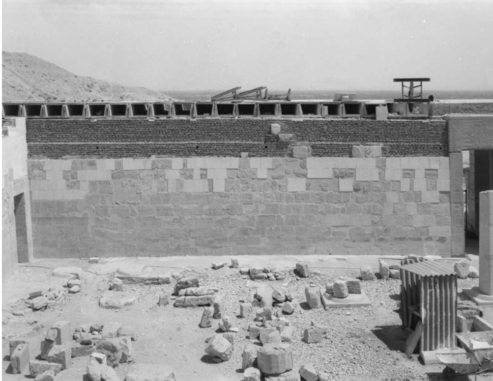
Fig. 34. View on the north wing of the east wall, season 1984/1985 (Courtesy of IMOC PAS, inv. no. DeB 1985_006_3).
